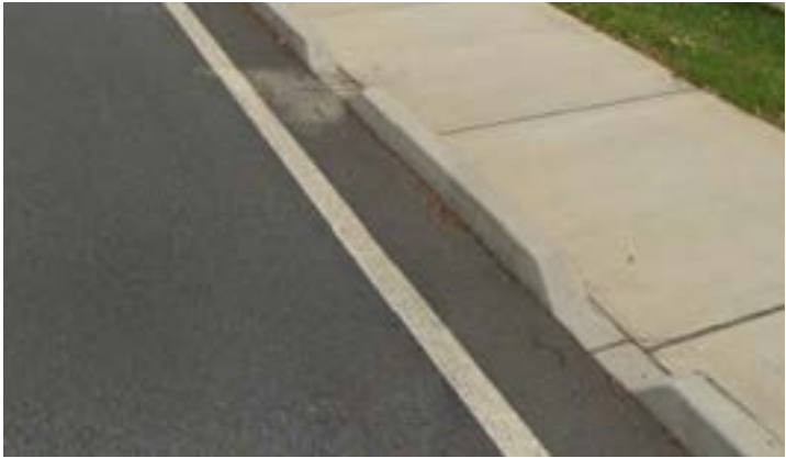
BROKEN KERB ALONG THE CHAPMANS ROAD TO PERMIT STORMWATER FLOW TO CENTRAL SWALE
